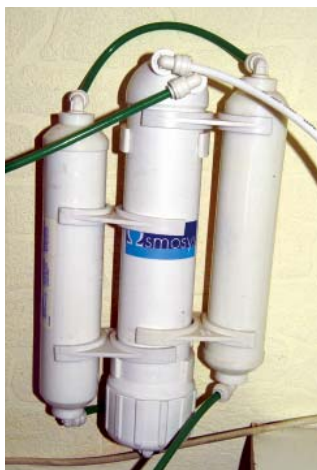
This reverse osmosis machine transforms water with a high ppm or EC into water with less than 10 ppm.
