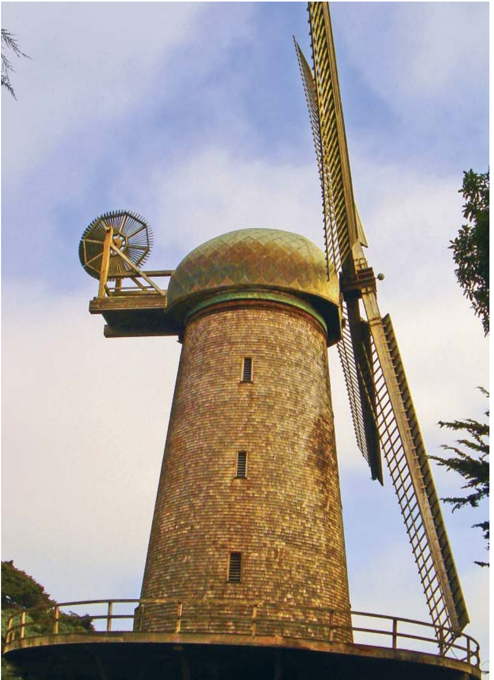
This air-powered windmill in San Francisco's Golden Gate Park has been pumping water to the gardens here for almost a century, without the use of any fossil fuels. Air has many uses!
